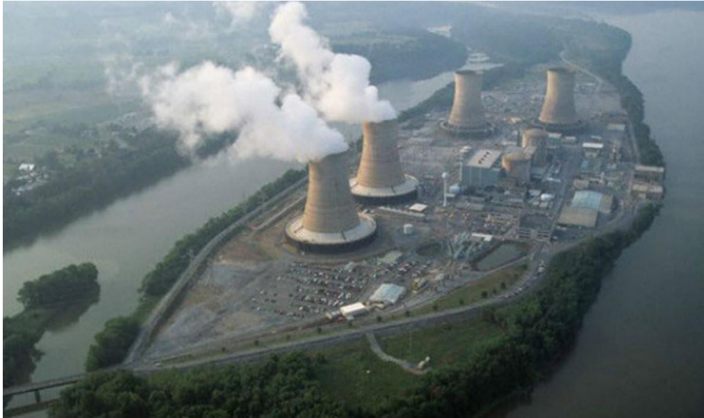
The Three Mile Island nuclear plant, shown above, is located on the Susquehanna River in Dauphin County. It shut down permanently in 2019.
